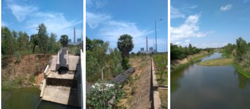
(Image: stormwater drain)
