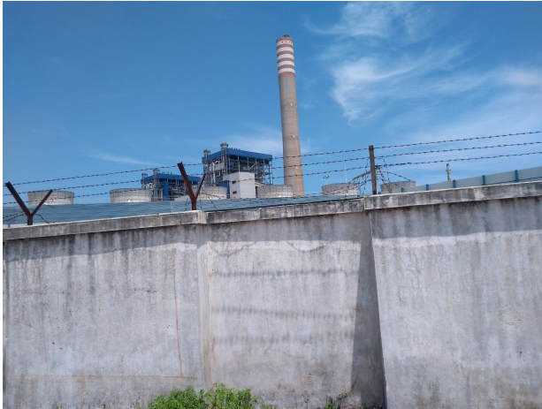
(Image: Top of the cooling tower)
