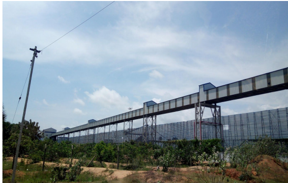
(Image: Coal conveyor belt)
