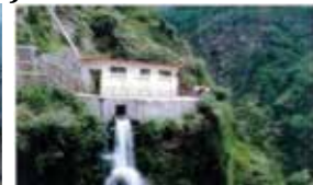
Small Scale Hydro Power Plant
