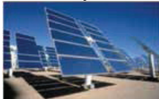
Solar Power Plant
