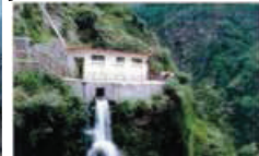
Small Scale Hydro Power Plant
