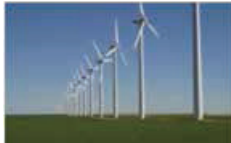
Wind Power Plant
