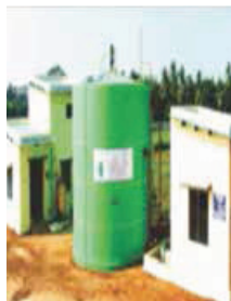
Distributed Biogas Plant
