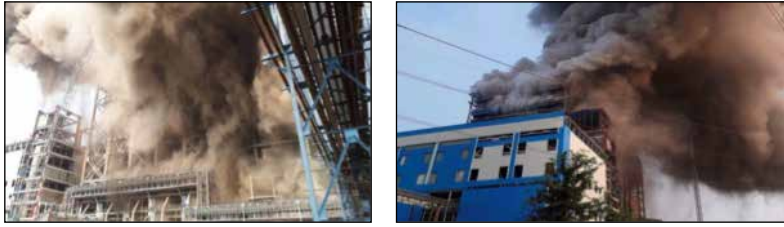
Pic 4.6: Furnace accident
