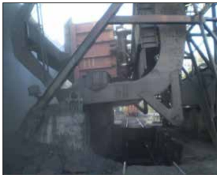
Pic 2.3: Wagon unloading
