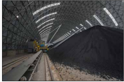
Pic 2.2: Closed stockpile
