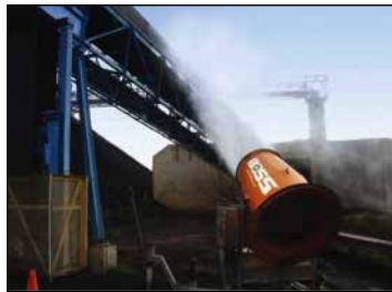
Pic 1.29: Water sprinkling on conveyors
