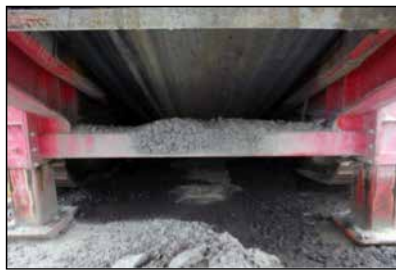
Pic 2.10: Coal wastage under conveyor
