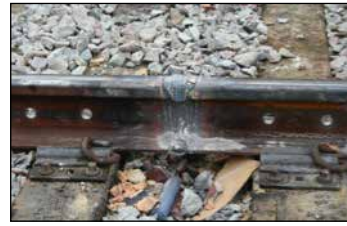
Pic 1.16: Welded Joints
