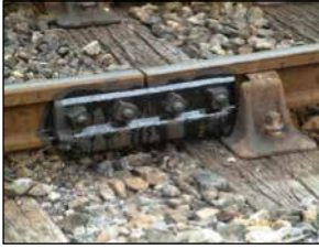
Pic 1.15: Bolted joints
