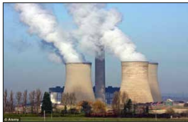
Pic 7.1: Cooling tower
