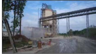
Pic 8.5: Fly ash silos
