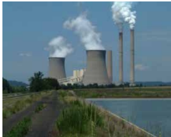
Pic 5.1: Flue gas from stack
